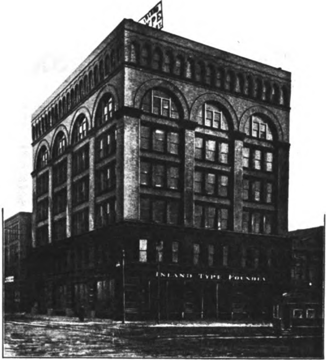
Saint Louis Office and Factory
